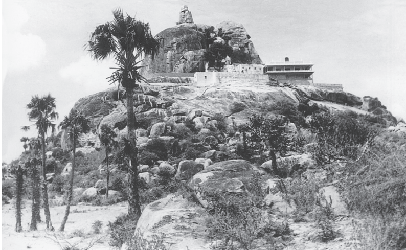
Photo showing completed construction work
